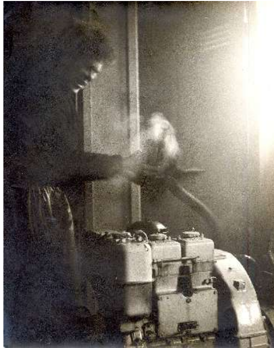
Lister Generator Exhaust
